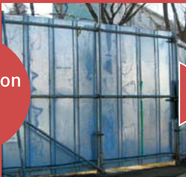
Set up Temporary Hoarding
